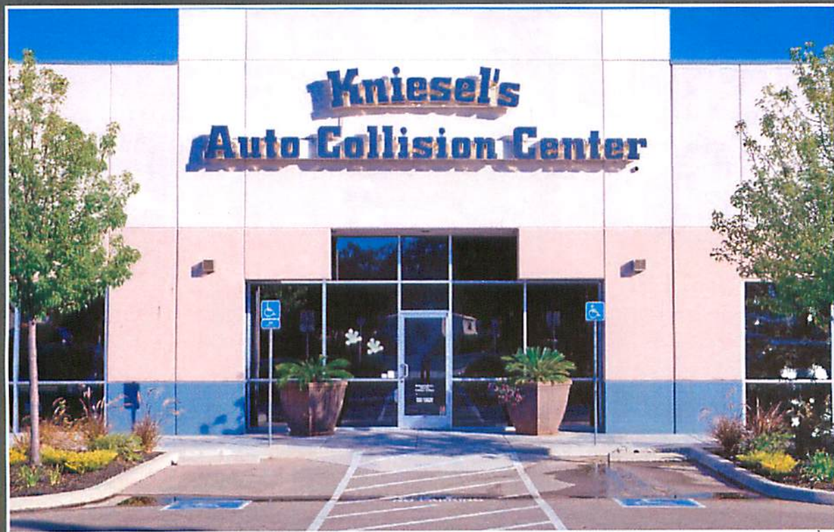
If it didn't say Kniesel's Auto Collision Center, you might mistake this building for a swanky office.
